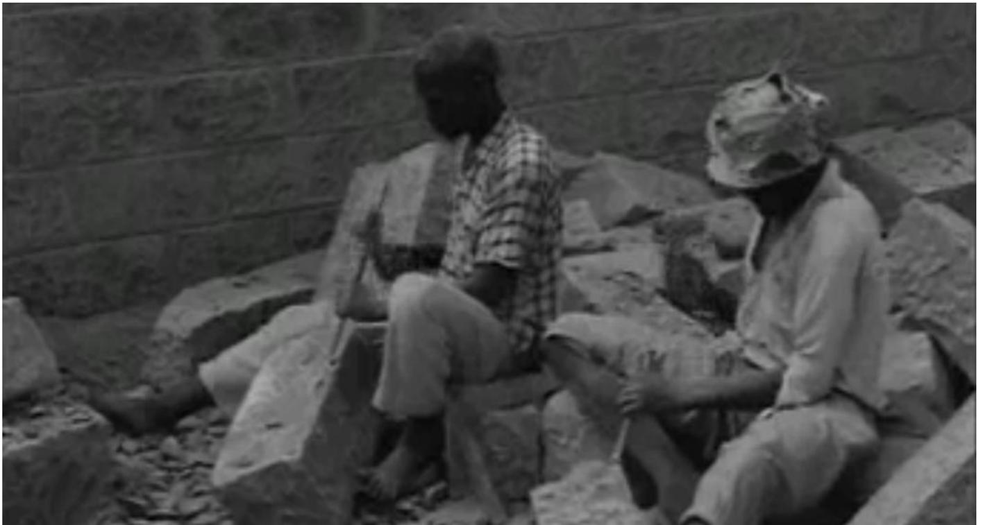
Indian foremen overseeing construction works. Skilled stone masons carving rocks to produce perfect shapes of solid stone bricks, a hallmark of construction material used in Kenya since the late 1800's
