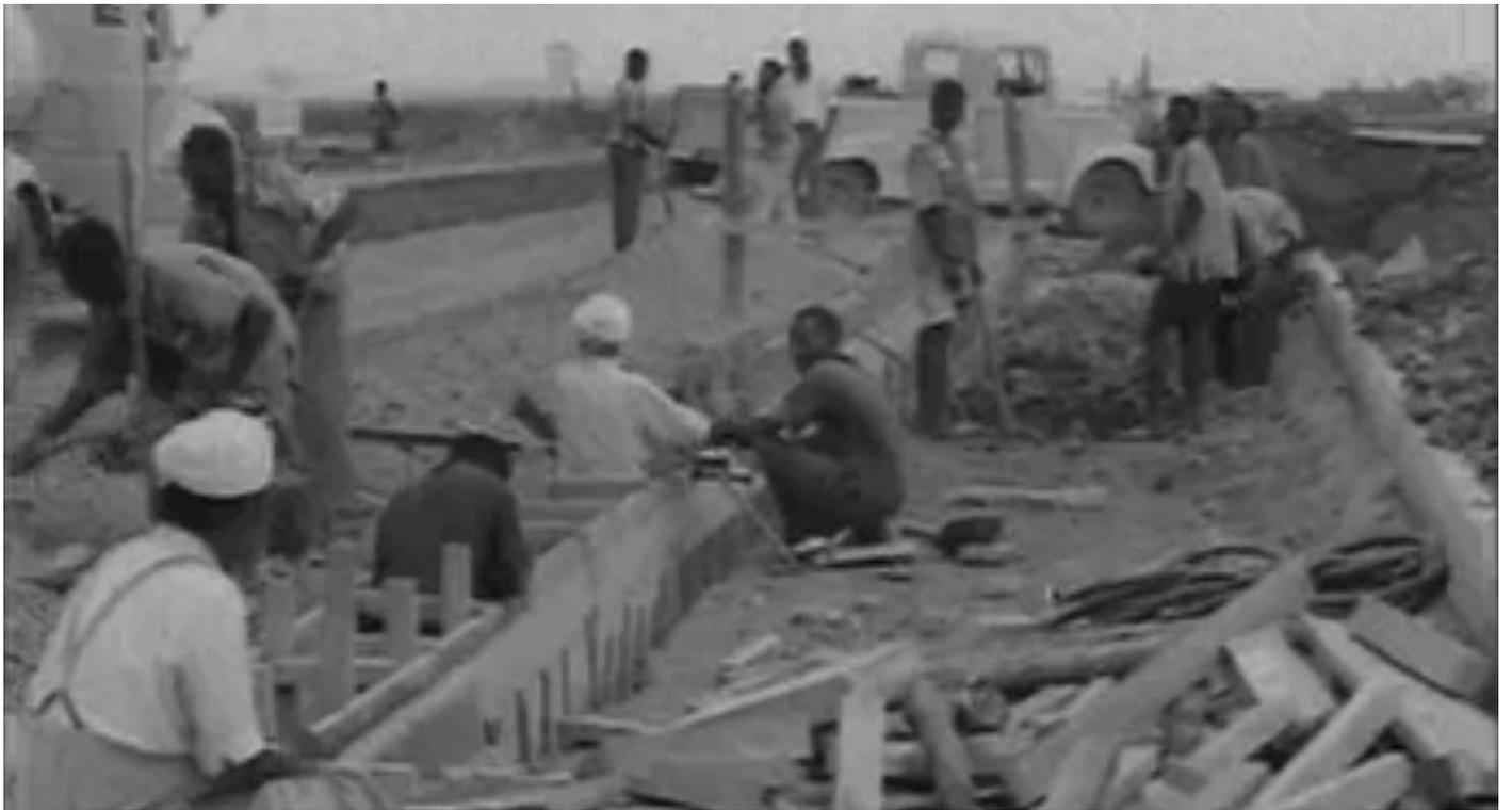
Skilled Sikh carpenters working on formwork for concrete ground beams and foundations.
